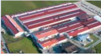
Plant I, Gremsdorf, Germany
