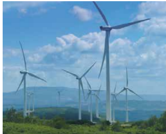
Onshore-windfarm: 3 MW turbines with rotor diameters of 90 m.
