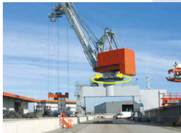
Harbour cranes, mobile harbour cranes
