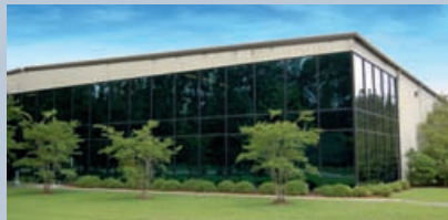
Plant III , Summerville, SC, USA
