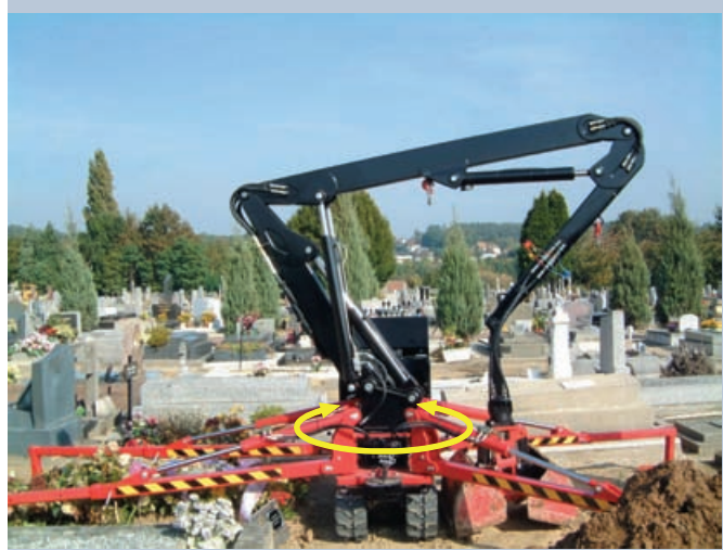
Cemetery excavator with the IMO Slew Drive WD-L 0343 .
